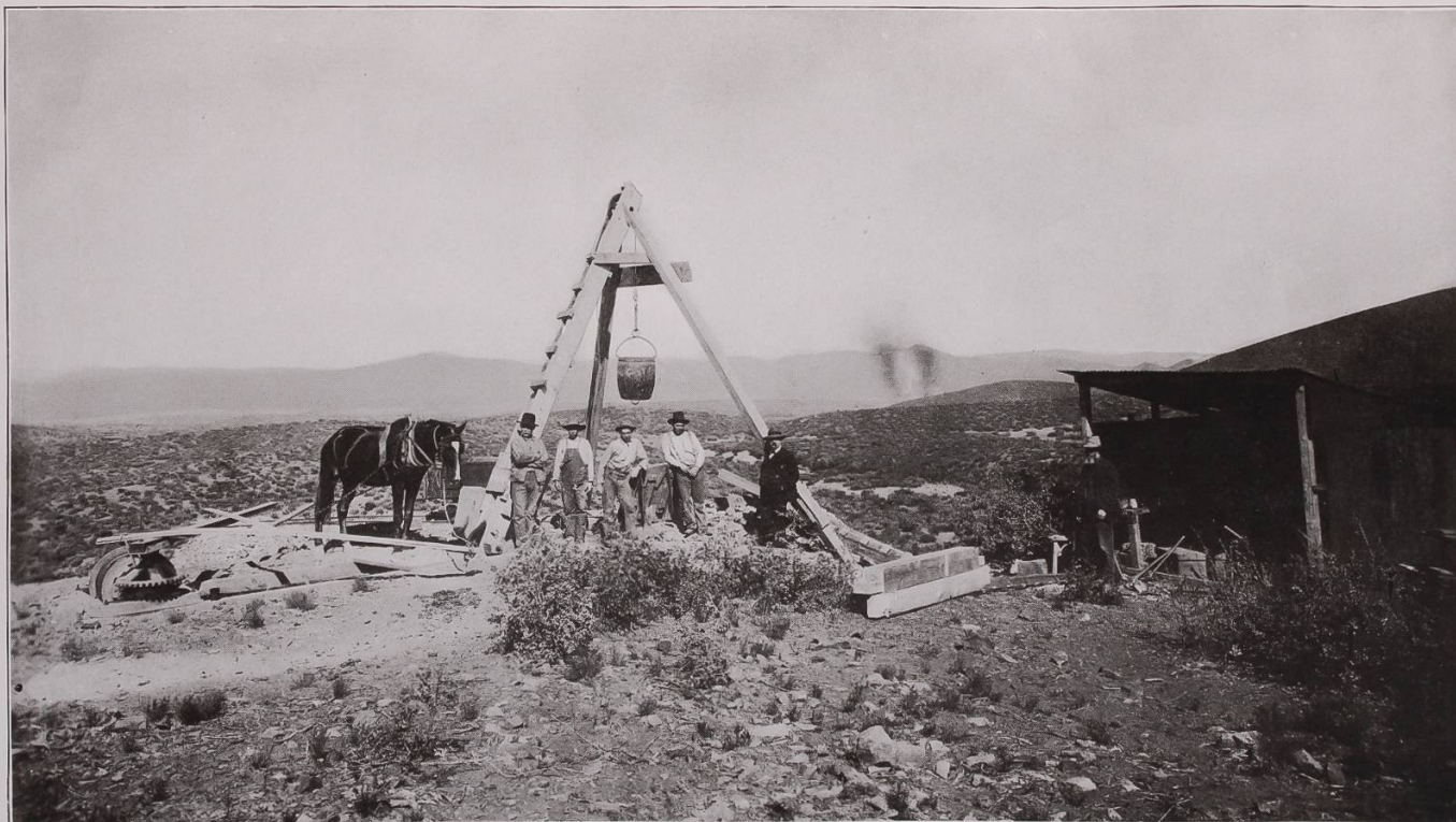
READ STAR MINE. SHOWING TRIPOD AND HORSE WHIM WHICH HAS SINCE BEEN REPLACED BY A FULLY EQUIPPED STEAM PLANT AS SHOWN IN PLATE VIII, MADE APRIL 17, 1907. SMOKE AT RIGHT OF TRIPOD SHOWS LOCATION OF THE ARIZONA SMELTING COMPANY AT HUMBOLDT.
